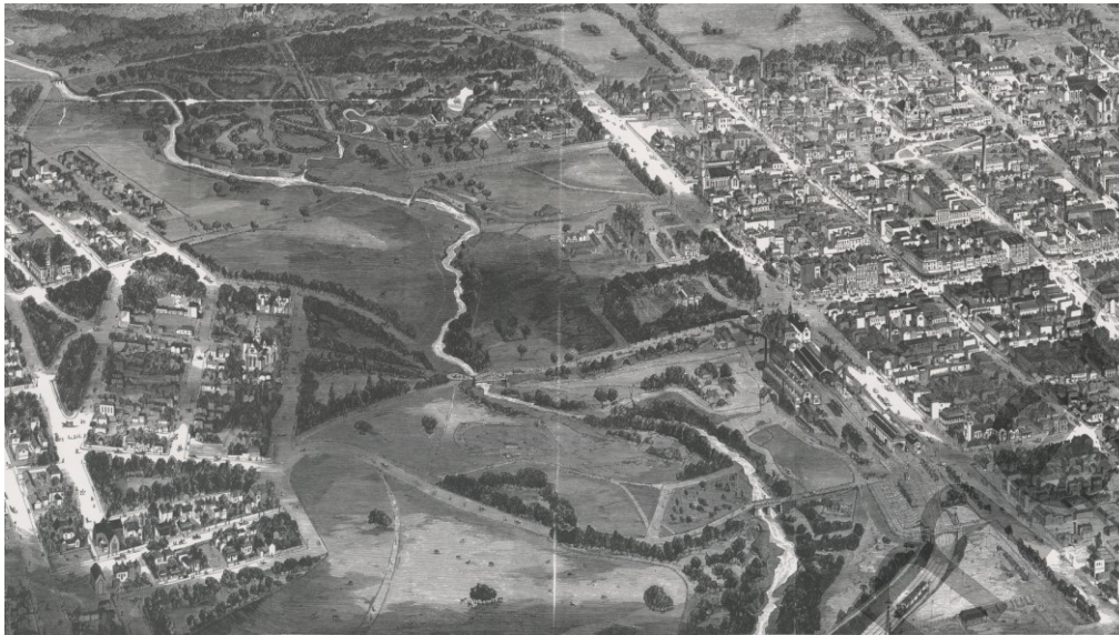
Figure 3: Section from: Facsimile of a bird's-eye view of Adelaide, from a point on Pennington Terrace, in 1876 "A capital view of the City of Adelaide", Cooke, A.C. (Albert Charles)
